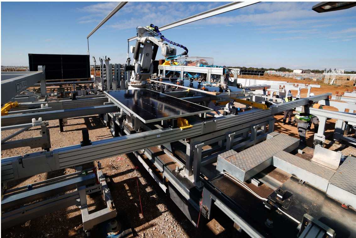
Figure 5.9.: An articulated robot handles PV modules using multi-purpose specialized grippers. Image credit: Daniel Mora
